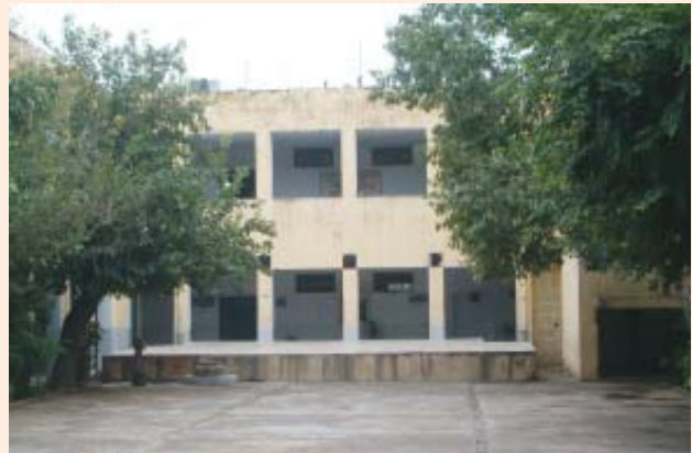
School Building at Ramesh Nagar (before retrofitting)
