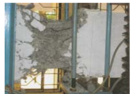
Fig. 18 Failure of Fibre Reinforced LRC Beam under High Shear
