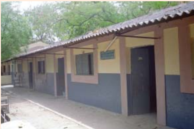
Vasant Vihar School Building after retrofitting
