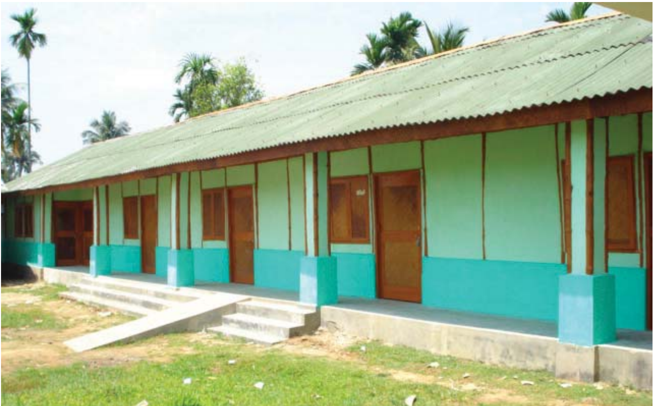
Construction of School Building in Tripura based on Bamboo based Technologies.
