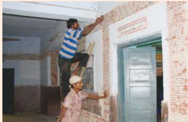
Fixing of WMM belt at lintel level
