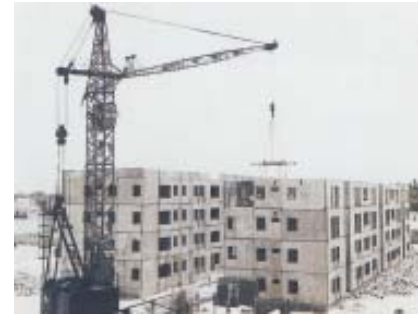
Fig. 2 Industrialised Building Construction
