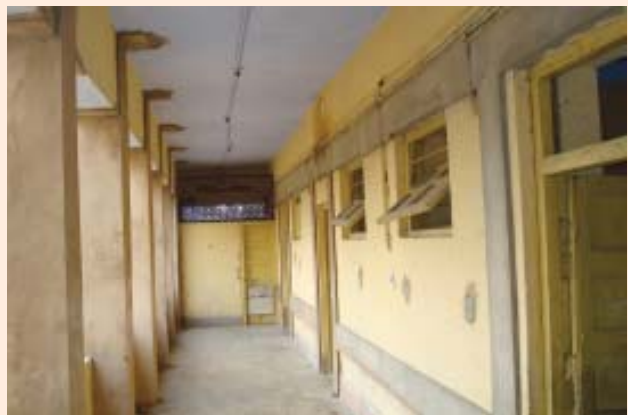
Completion of lintel level belt and encasement of columns
