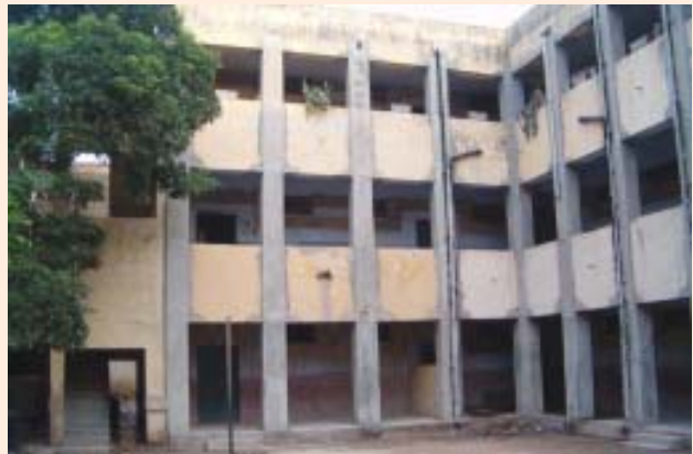
Ram Nagar School Building after retrofitting
