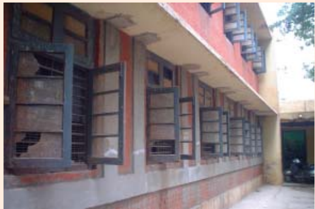
Encasing of windows and horizontal belt at sill level
