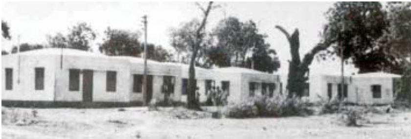
A Row of Houses Constructed using Moveable Formwork
