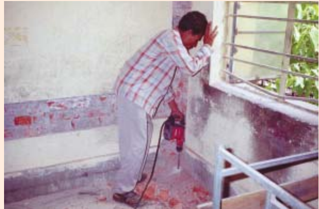
Drilling of hole for vertical corner reinforcement
