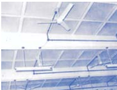
Fig. 3 Waffle Shell Roof System
