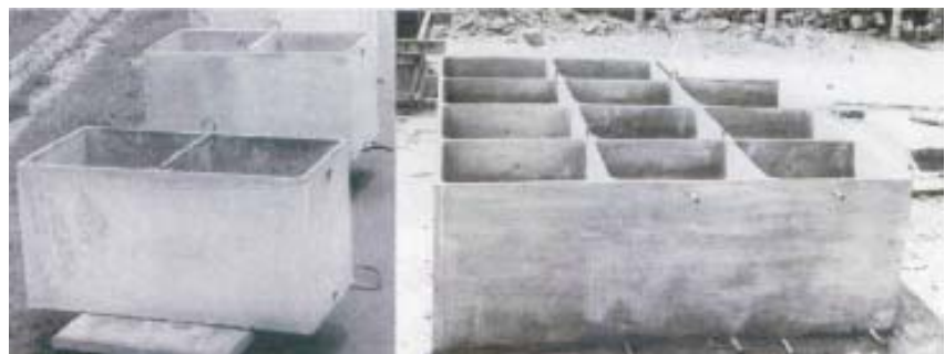
Fig. 5 (a) Multi-Cellular Water Tank
