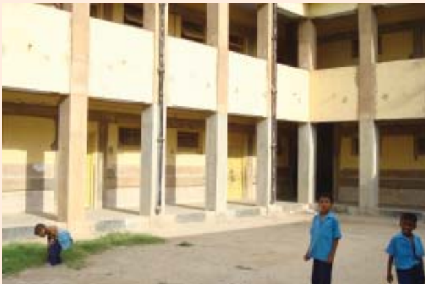
Rana Pratap Bagh School Building after retrofitting
