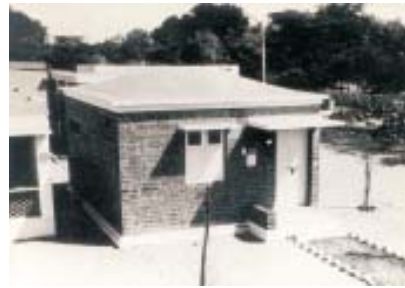
Independent House using Brick Funicular Shell
