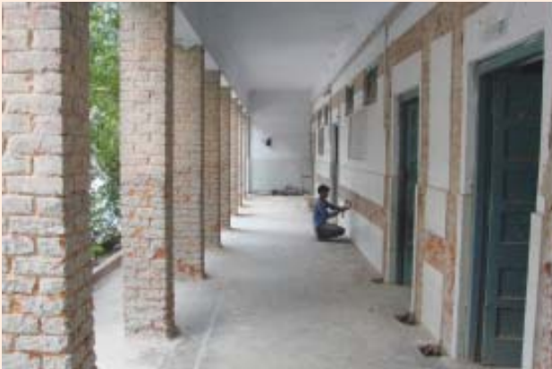
Removal of mortar for horizontal belt and encasement
