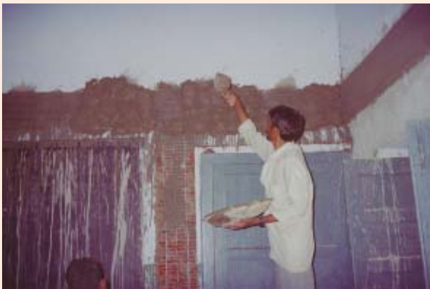
Plastering of WMM belt at lintel level
