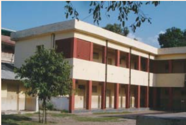
School Building at Rana Pratap Bagh (before retrofitting)
