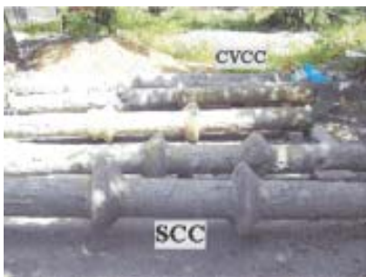
Fig. 15. Exhumed Under-Reamed Piles
