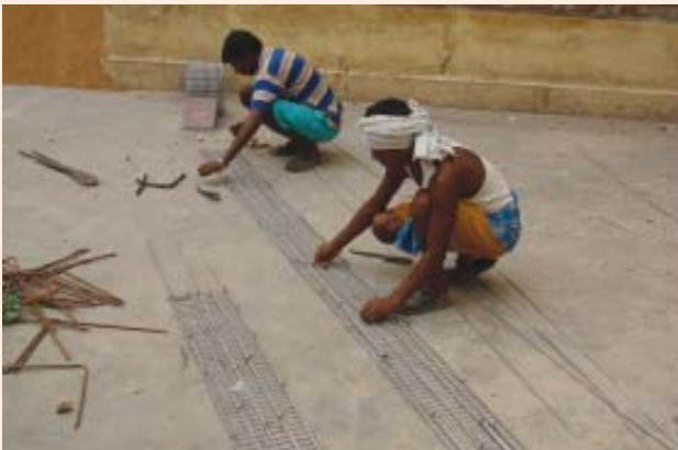
Fabrication of belt with WMM & Galvanized bars.
