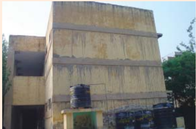
Ramesh Nagar School Building after retrofitting
