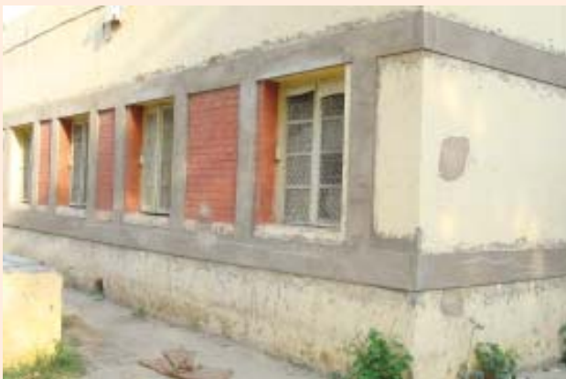
Window encasement with horizontal belt at sill and lintel level
