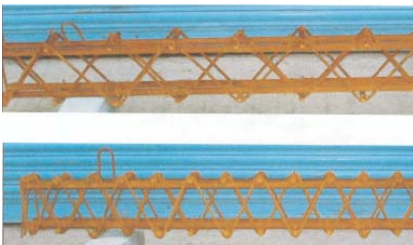
Fig. 17 Laced Reinforced Concrete Beams
