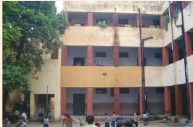
School Building at Ram Nagar (before retrofitting)
