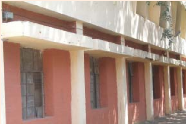
School Building at Sarai Rohilla (before retrofitting)
