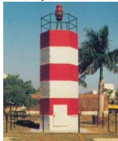
Fig. 10 Light Beacon Tower made using Polymer Impregnated Ferrocement Panels
