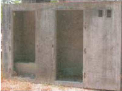
Fig. 6(a) Single Service Core Unit
