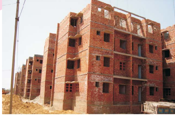
Brick Load Bearing Construction
