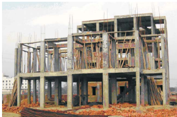
RCC Framed Construction
